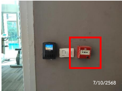
Fire Alarm Manual Call Point
