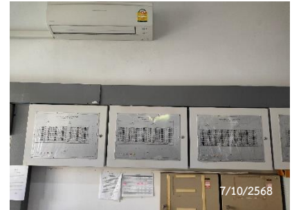
Graphic Annunciator Fire Alarm System
