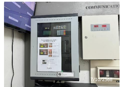
Fire Alarm Control Panel
